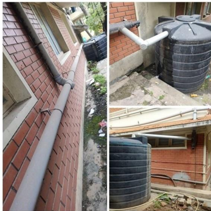
Figure 4-9: Rain water harvesting system
