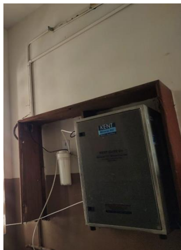
Figure 4-6: RO water purifier
