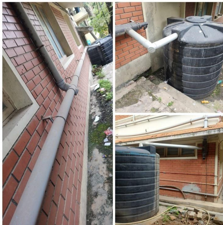
Figure 4-5: Rain water storage system and tanks
