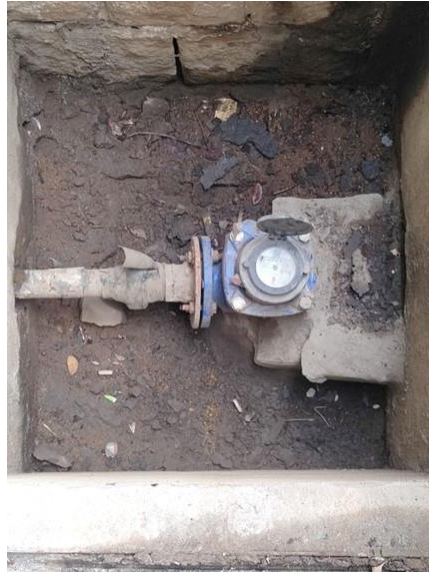
Figure 4-11: BWSSB water flow meter
