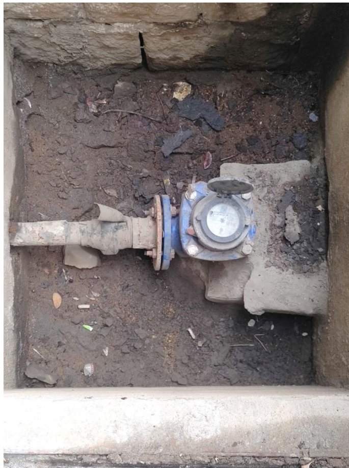
Figure 4-1: Water flow meter
