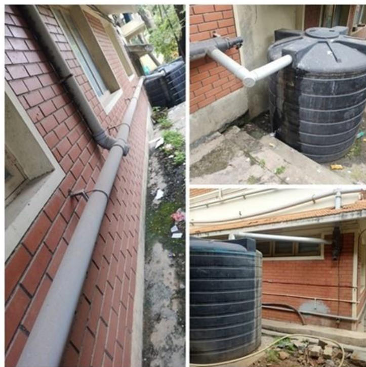
Figure 8-3: Rain water harvesting system
