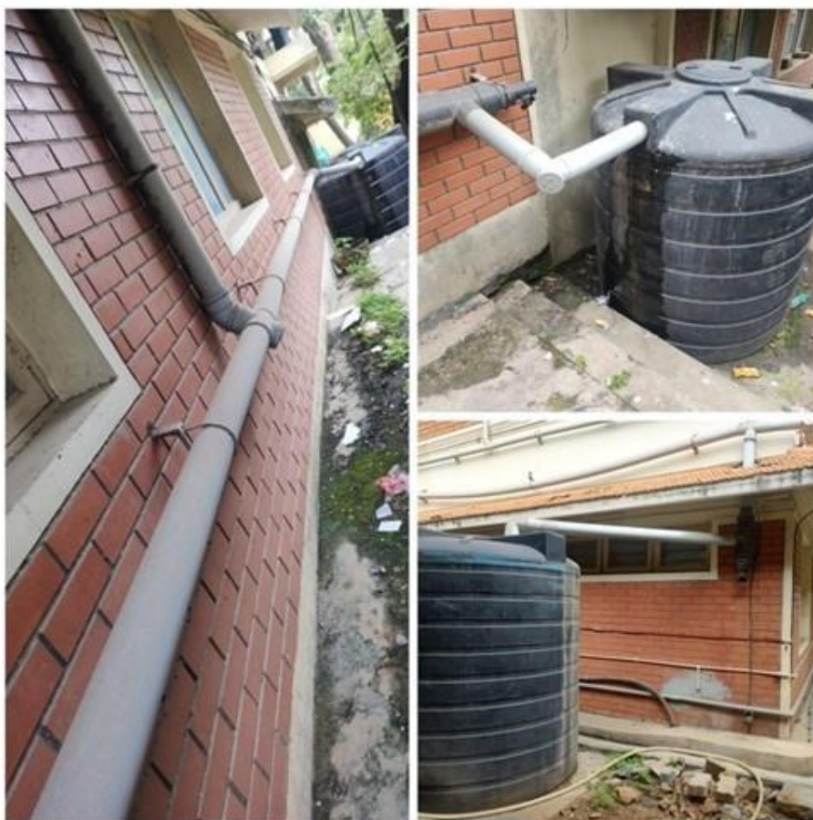
Figure 4-7: Rain water harvesting system
