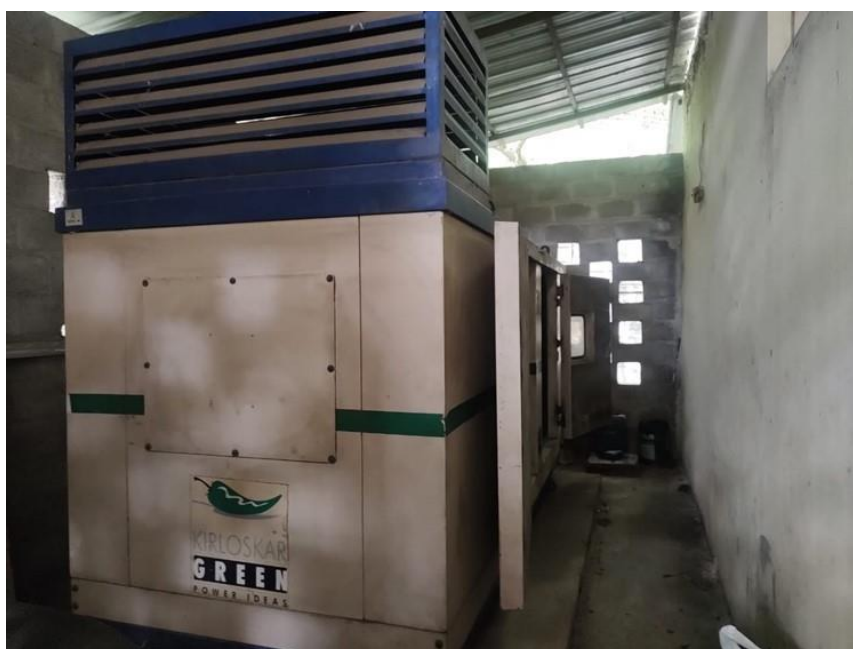
Figure 5-2: Diesel Generator (DG) Set
